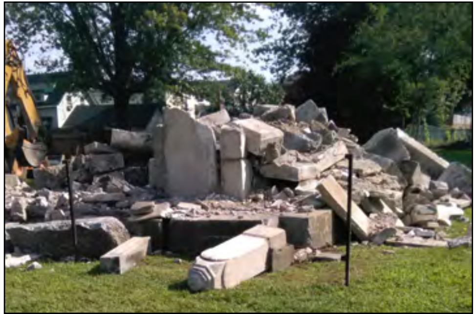
The immediate aftermath of the wrecking crew's first pass on the morning of 14 August 2017. (Source: Barrie Brown)
